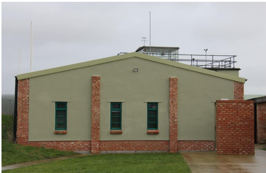
New exhibition hall with blast wall
