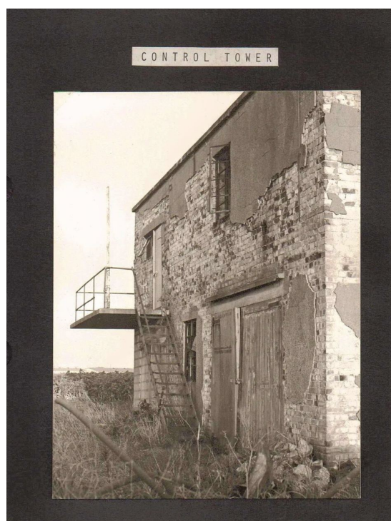
The dilapidated Control Tower, with the double doors that Percy Kindred cut into the walls
