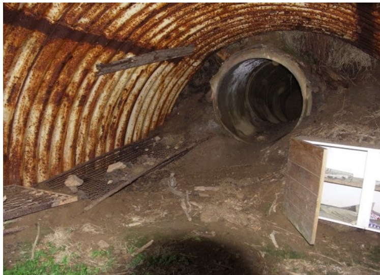
Inside the Grange Patrol Operational Base
