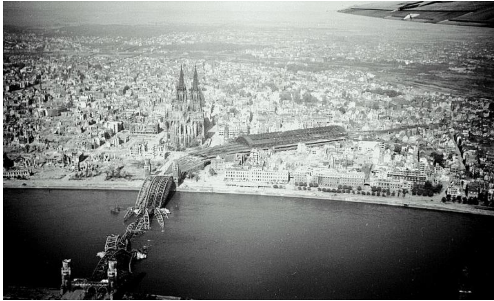
Cologne Cathedral. Damage can be seen In the city.
